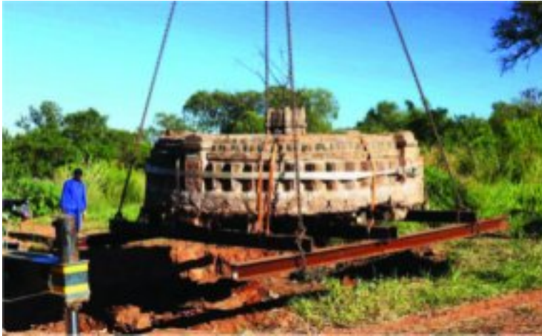
Lifting the fountain
