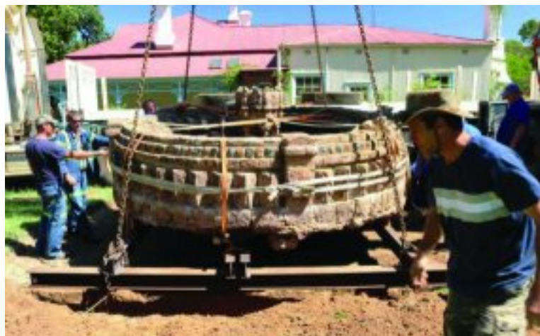
Installing the fountain in the garden at the McHardy House Museum
